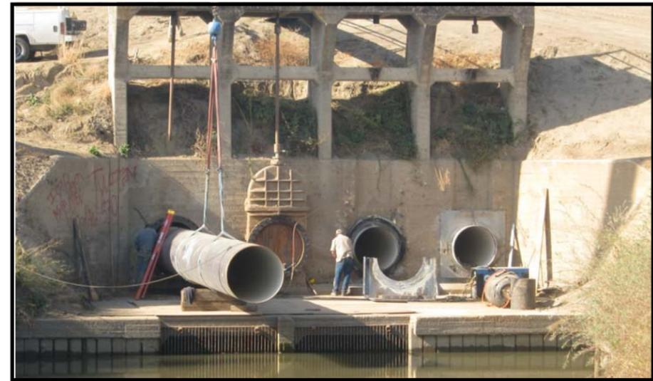
Sleeving a 48 inch Pipe Inside Old 54 inch Pipe Through the River Levee
